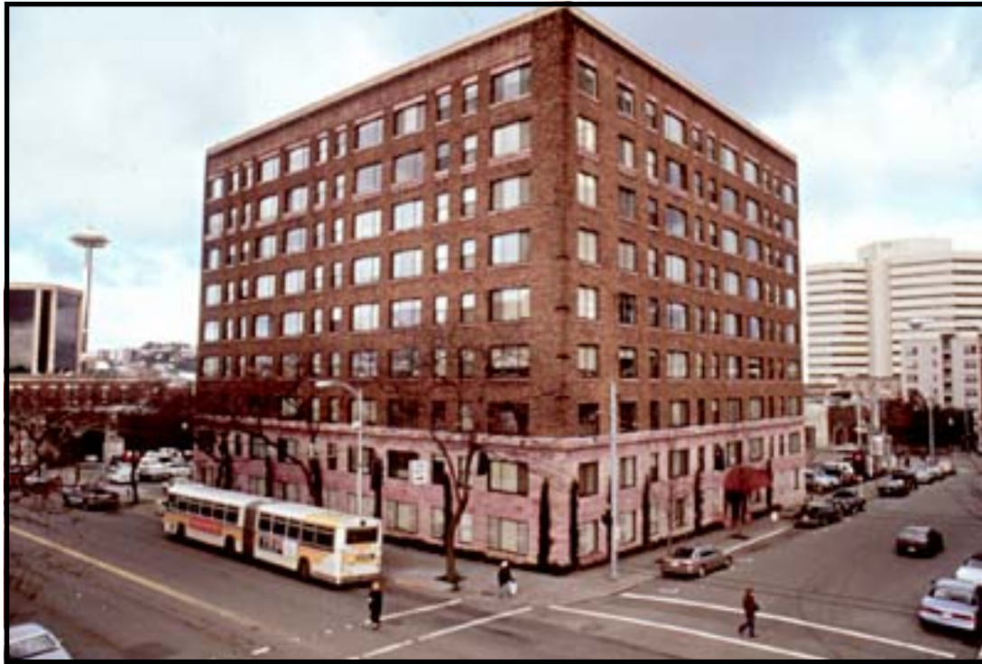
The Cornelius Apartments 306 Blanchard Street, Seattle, WA 98121
