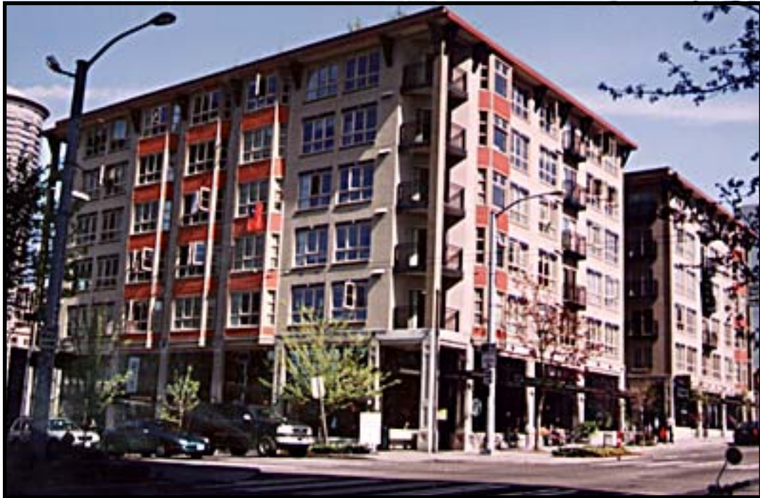
The Lenora Apartments 211 Lenora Street, Seattle, WA 98121
